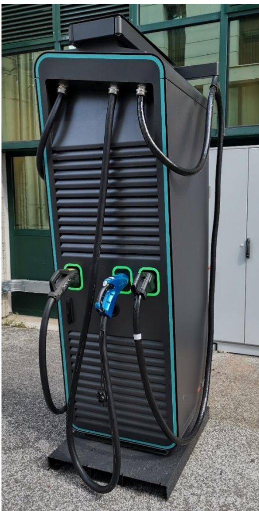
Figure 14: Fully installed cable management HYC300
