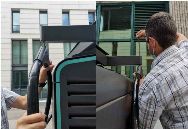
Figure 13: Fastening the cable holder to the cable management arm
